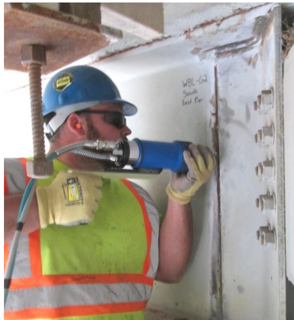
Figure 1. Ultrasonic impact treatment (UIT/UP) of welded elements of a highway bridge
